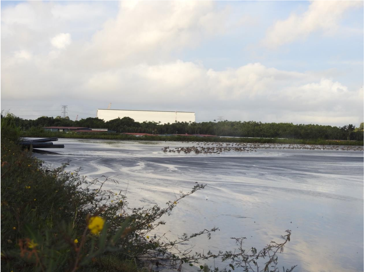
Photo 15. Sejingskat Ash Pond (Credit: Batrisyia Teepol).
