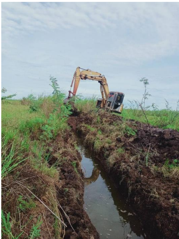
Photograph 6. Contractor infilling redundant ditches (Task D)
