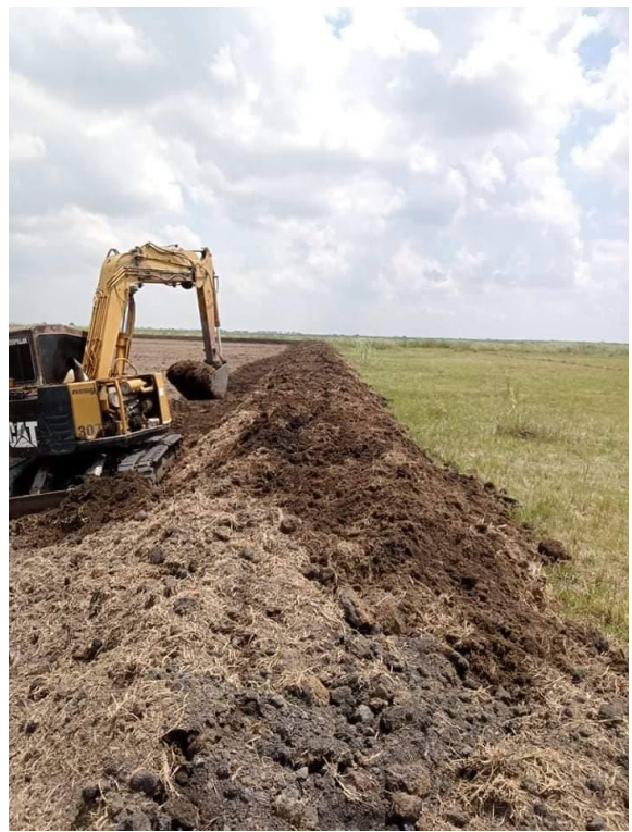
Photograph 7. Construction of the bund to retain water (Task B)
