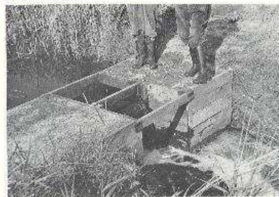
Fig. 5. An early-made wooden sluiceway to restrict the flow of water from a series of drainage canals (the Sluiceway) to the water level in the Swamp at a certain point, to allow the water to be used for the Swamp. (Photo: M. J. Axell)
