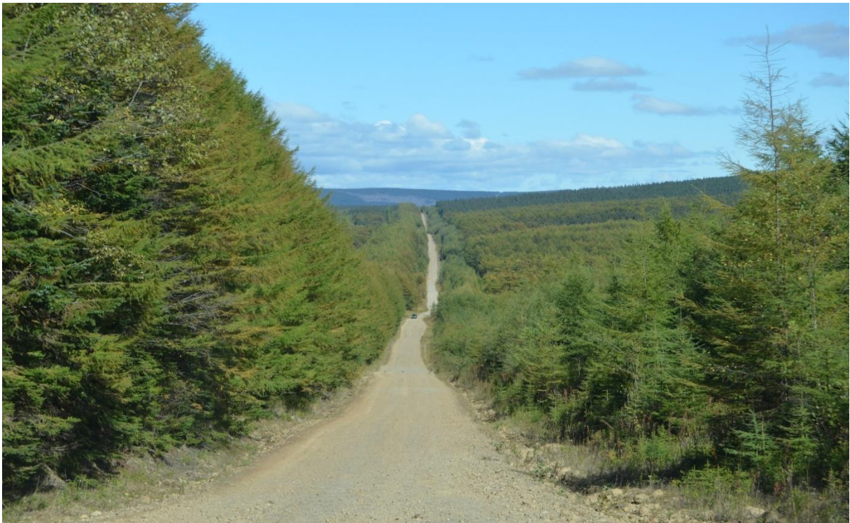
Figure 9: The bulk of regional roads are fortified embankments that require constant repair due to high precipitation
