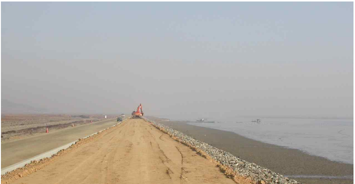
Figure 15. Construction of the inner dyke. Hwaseong Wetlands, January 2008.
